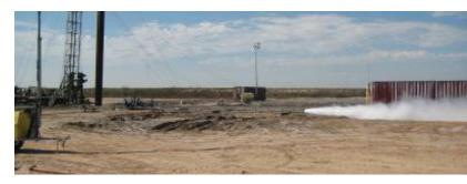
The blowout recovery phase of the project required rigging up a snubbing unit, for fishing operations and running a kill string. During the rig up phase, production equipment was set up to produce the gas on emergency sales, until the kill was completed. Initial plans were made to locate the tubing fish, latch the fish and pump the kill through the kill string and fish.
